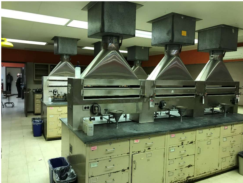
Photo 6 - Laboratory exhaust units (installation date not known) that are not associated with a fume hood located within the Natural Science Building.
