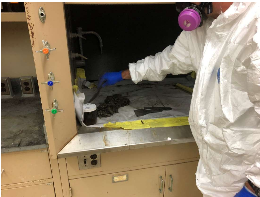
Photo 10 – Collection of dust/debris from within the duct of one of the fume hoods in the General Chemistry Laboratory.
