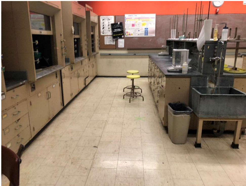
Photo 3 – Original fume hood units (circa 1972) located within the General Chemistry Laboratory.
