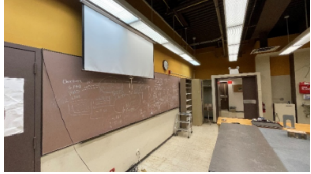
View in Room #2044 Along North Wall
