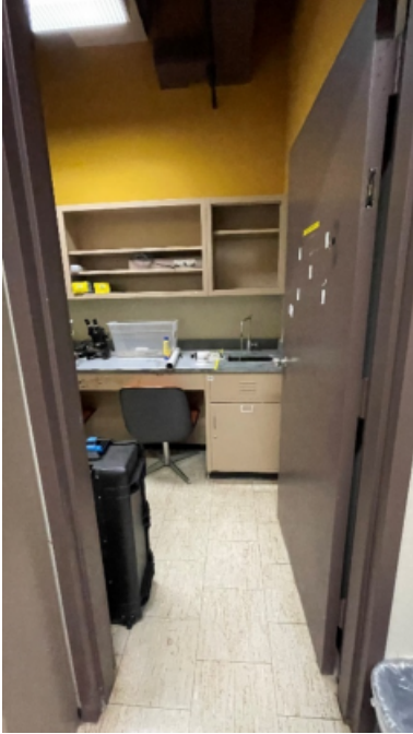
View in Room #2035 from Doorway
