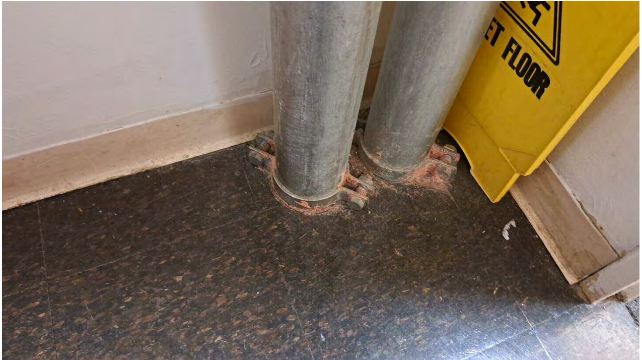
Potential new riser location. Tile is negative, but mastic is positive for asbestos.
