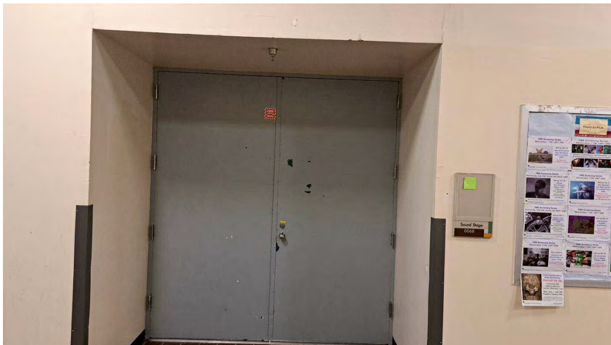
Above is another typical door that tested positive for lead on the doors and casings in Music
