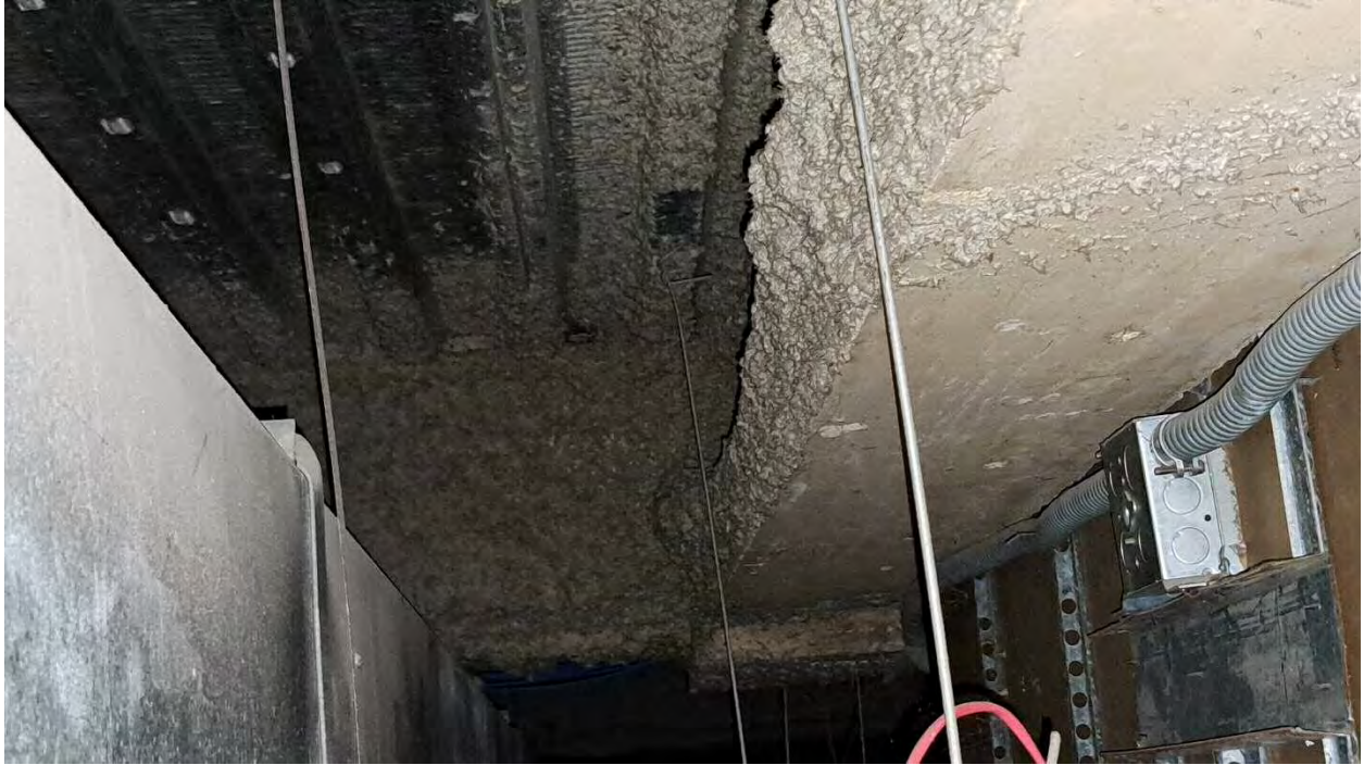
Typical visual arts above ceiling conditions and typical fireproofing to be treated as asbestos
