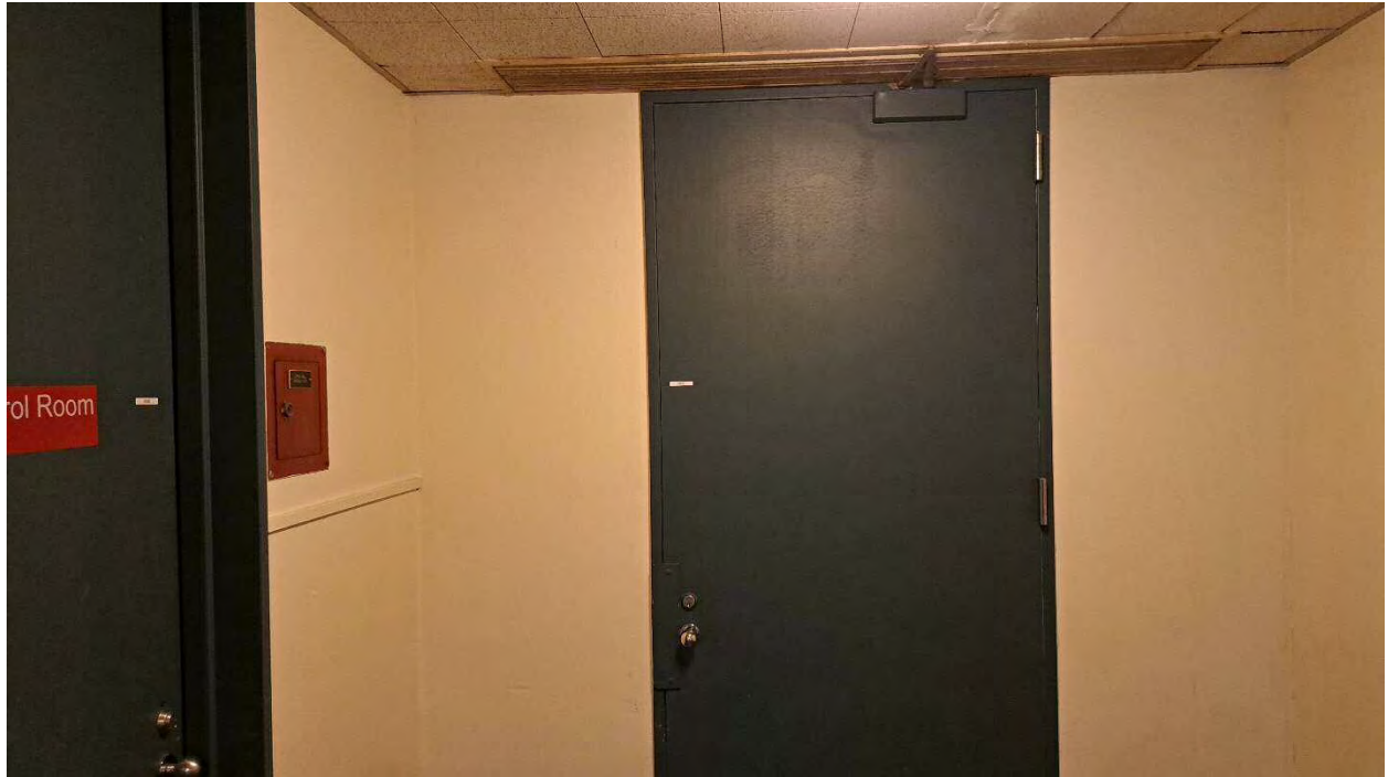
More typical doors that tested positive for lead on the doors and casings in Music
