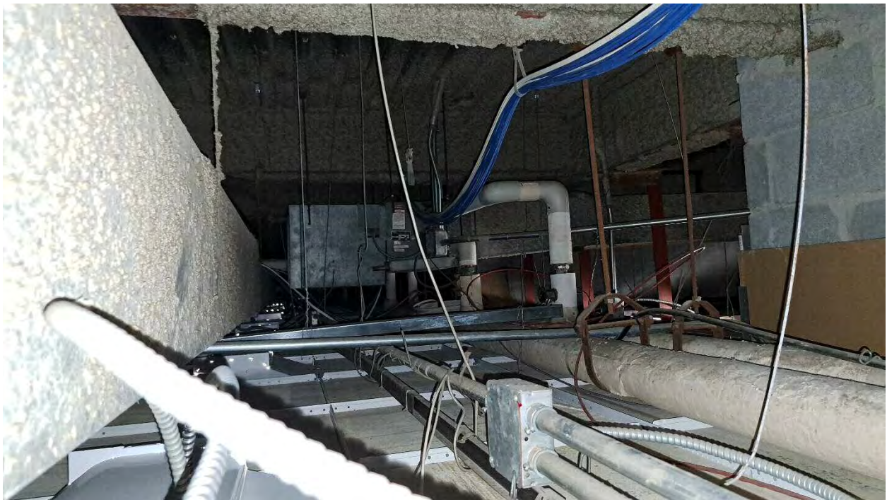
Potential new riser location. Tile is negative, but mastic is positive for asbestos.
