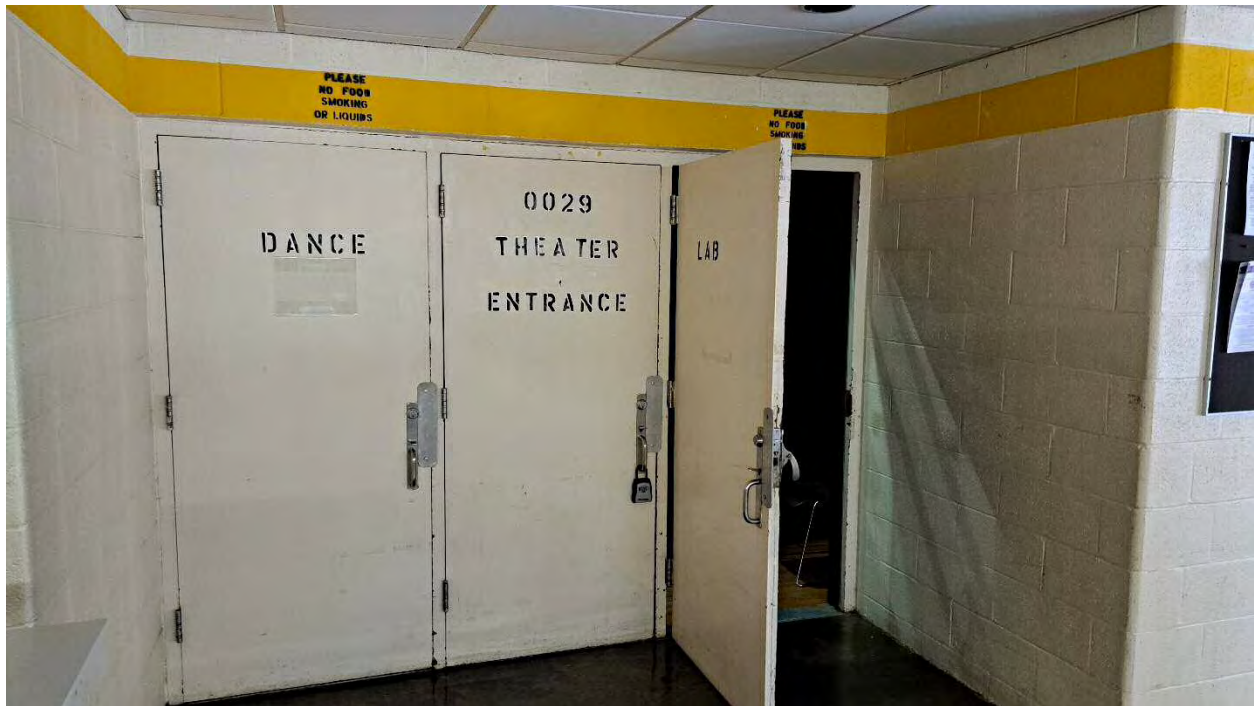
Another set of doors that tested positive for lead paint.
