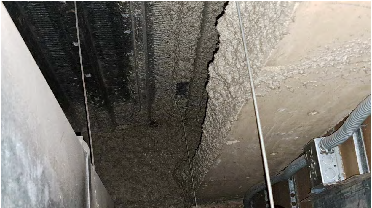
Typical visual arts above ceiling conditions and typical fireproofing to be treated as asbestos
