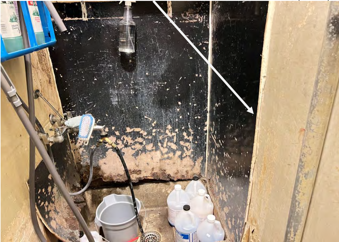
ABOVE: COMMUNITY CENTER SOUTH – NYPIRG OFFICE – ACM FLOOR TILE MASTIC BELOW: COMMUNITY CENTER SOUTH – CUSTODIAL CLOSET – ACM CAULK (WHITE)
