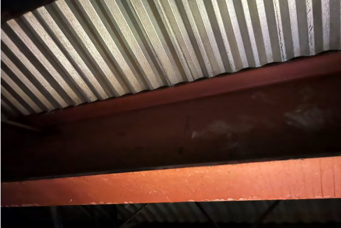
ABOVE: Community Center South, Throughout – LBP Support Beams
