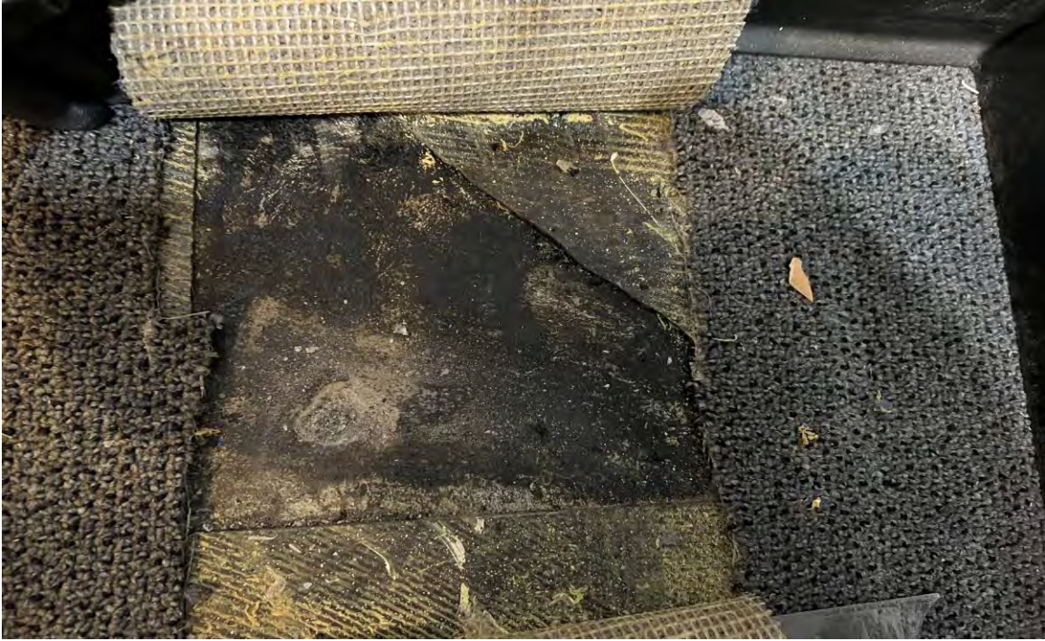
ABOVE: COMMUNITY CENTER SOUTH – NYPIRG OFFICE – ACM FLOOR TILE MASTIC BELOW: COMMUNITY CENTER SOUTH – CUSTODIAL CLOSET – ACM CAULK (WHITE)
