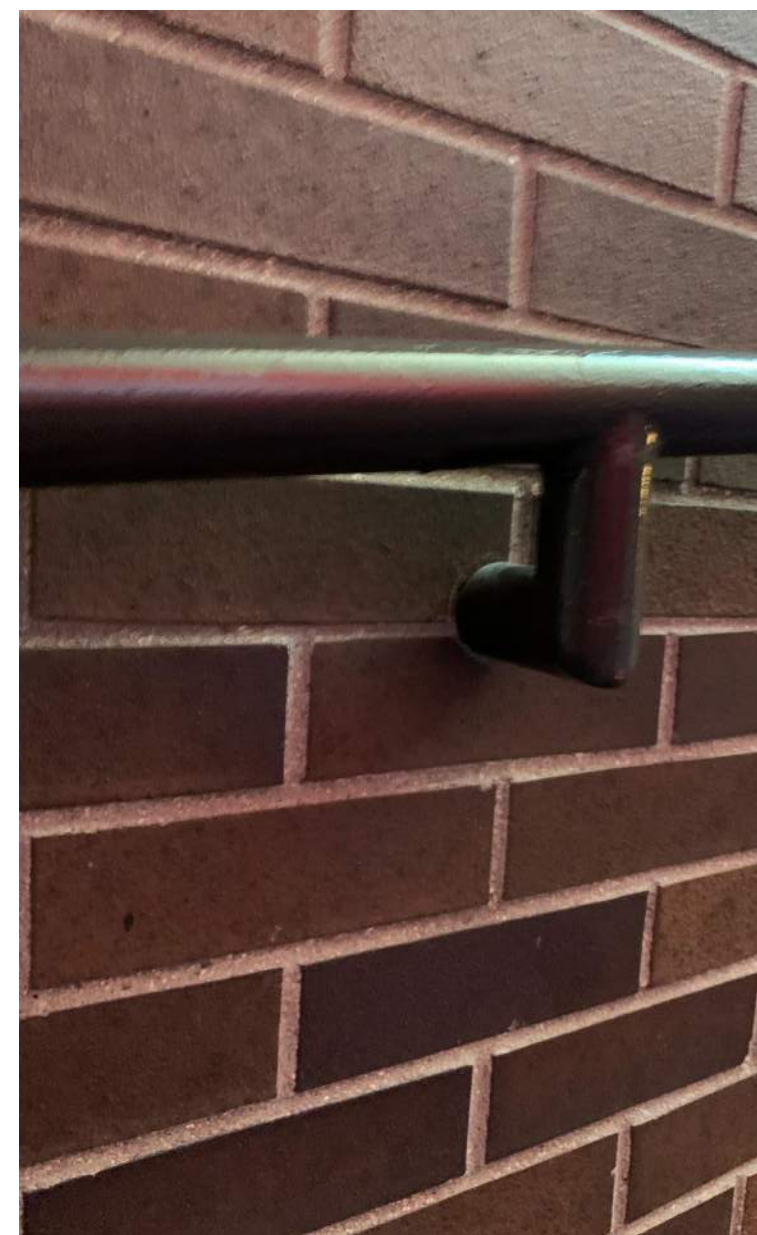
TYPICAL HANDRAIL CONNECTION
