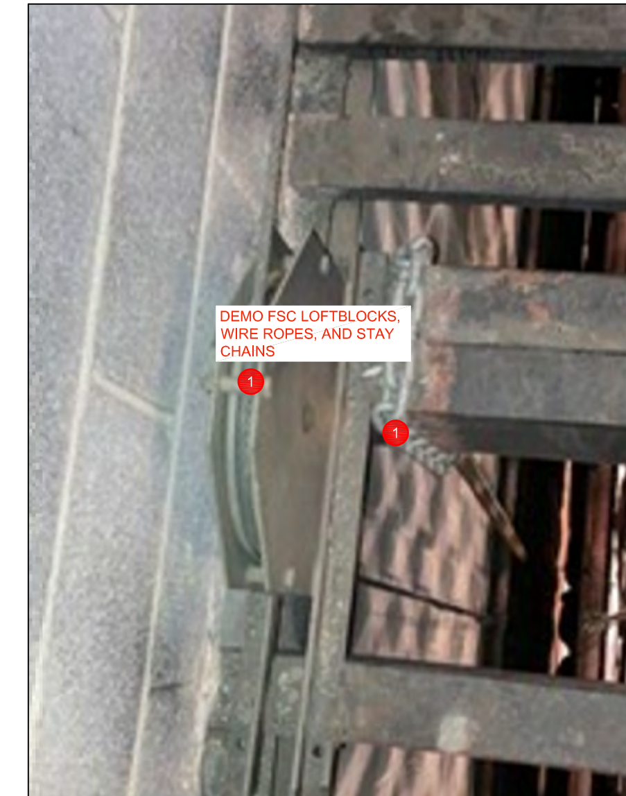
3 GRID LEVEL FSC RIGGING NTS
