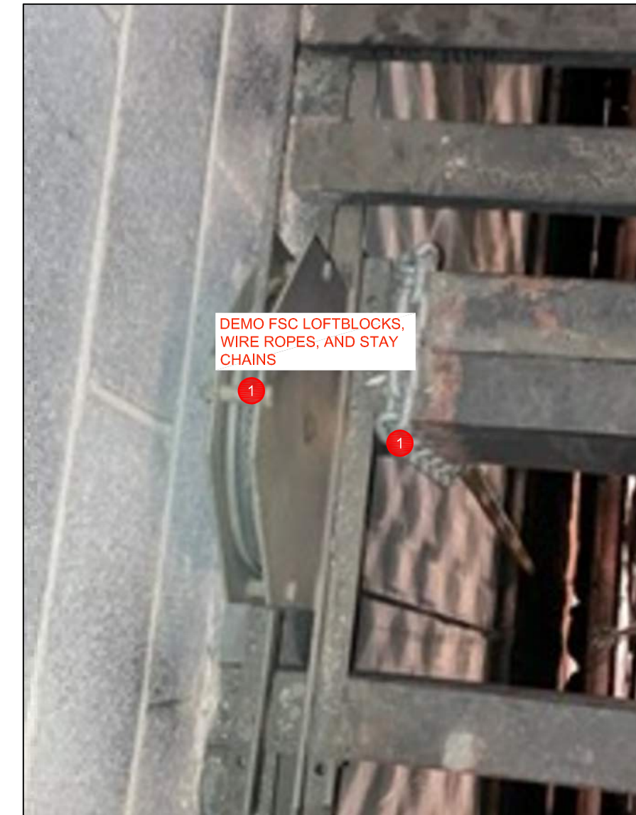
3 GRID LEVEL FSC RIGGING NTS
