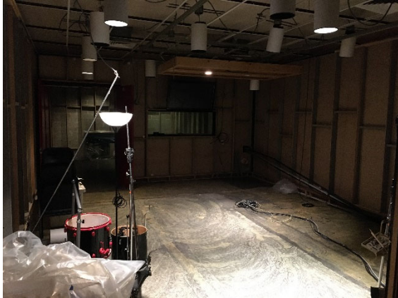
View of Room #1007 Looking Southeast
