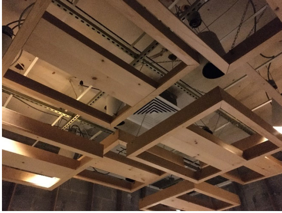
View of Room #1007A Ceiling
