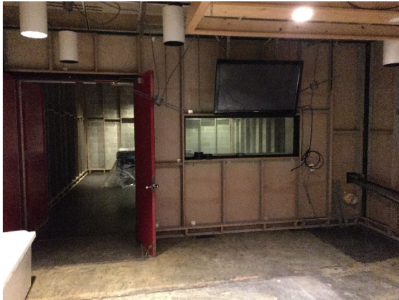
View of Room #1007 at Separation Wall
