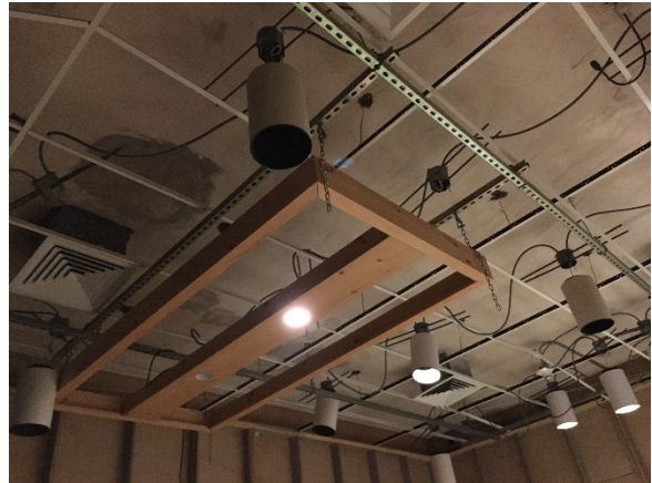
View of Room #1007 Ceiling
