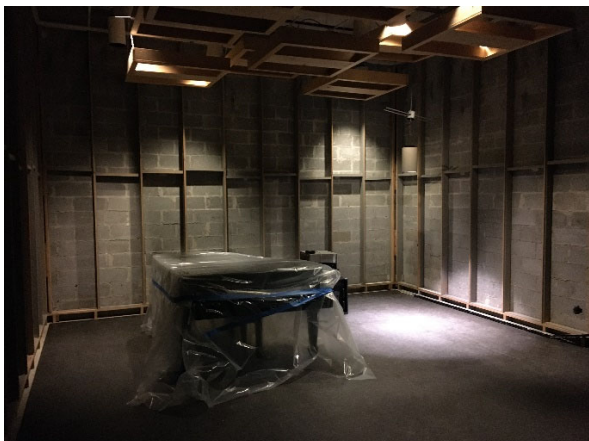
View of Room #1007A Looking Southeast
