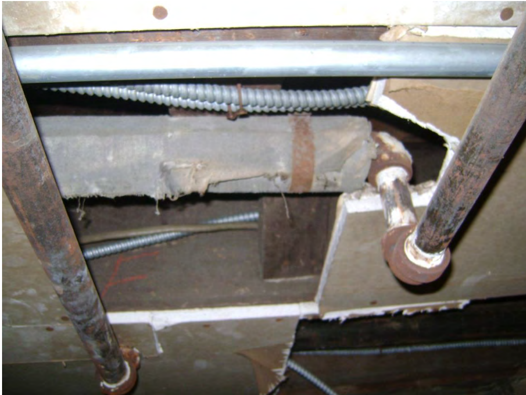
Sample #154 - Pipe Insulation - 22.20% Chrysotile
