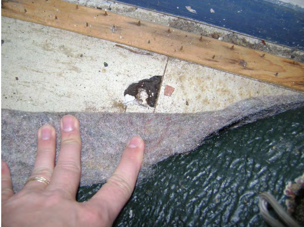
Sample #216 – Floor Tile – Beige with Streaks – 1.4% Chrysotile
