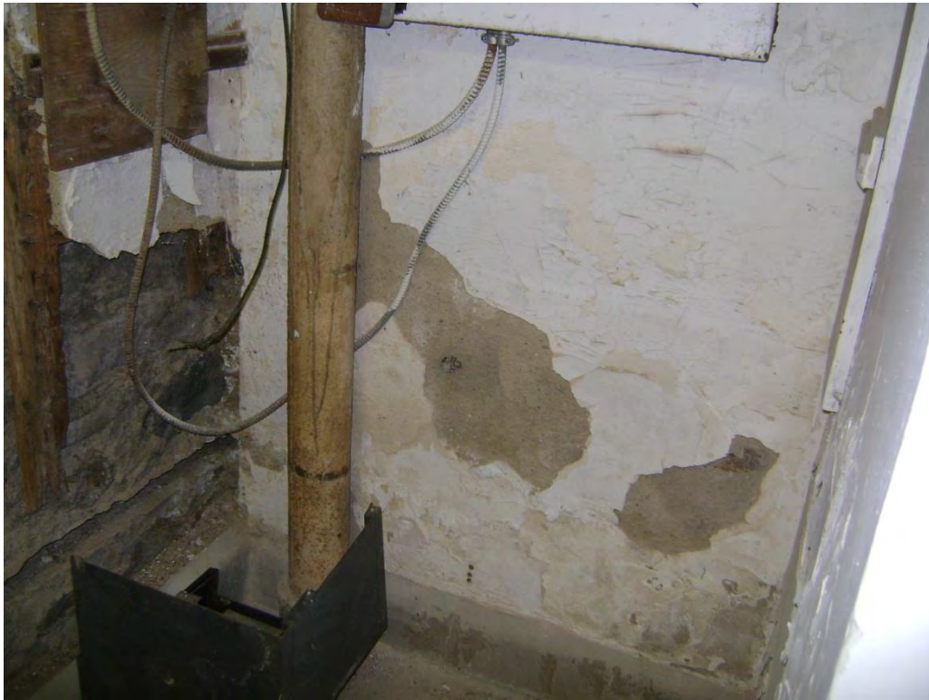
Sample #10 – Plaster Wall Base Coat – 1.48% Chrysotile
