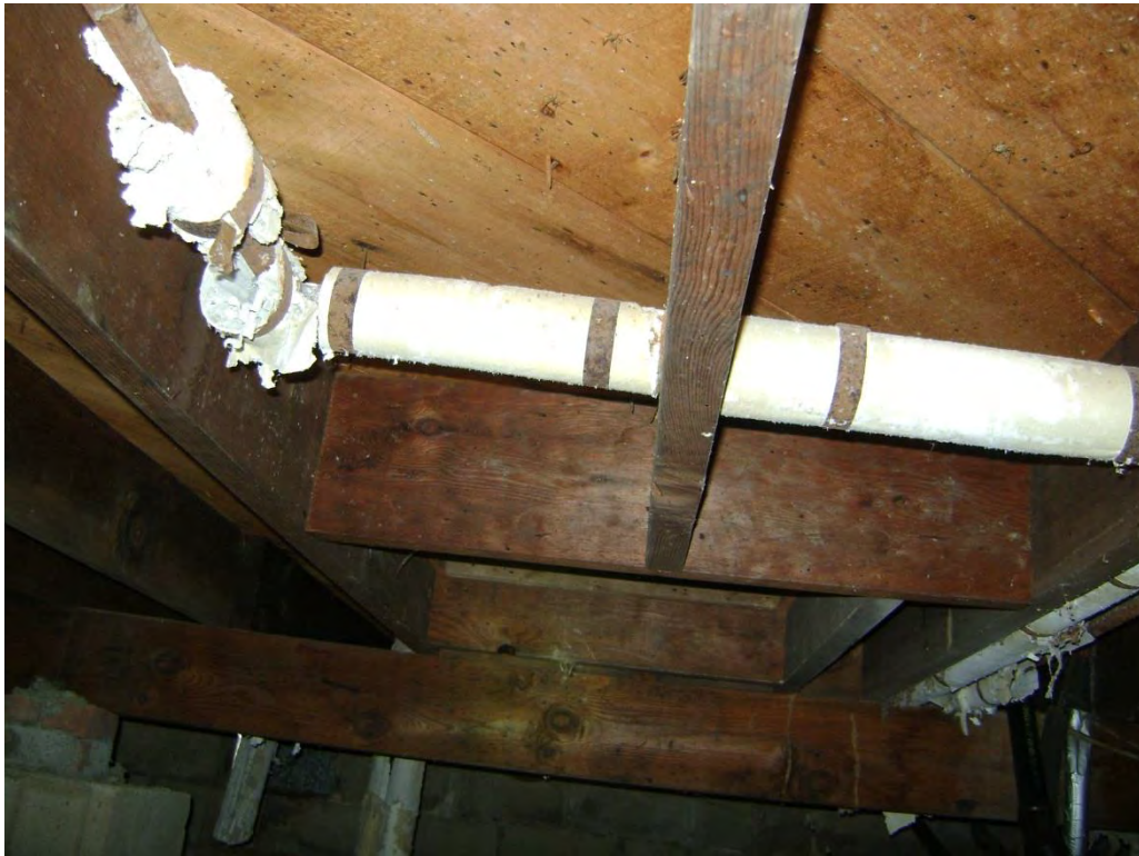
Sample #250 – Pipe Insulation – 50.00% Chrysotile
