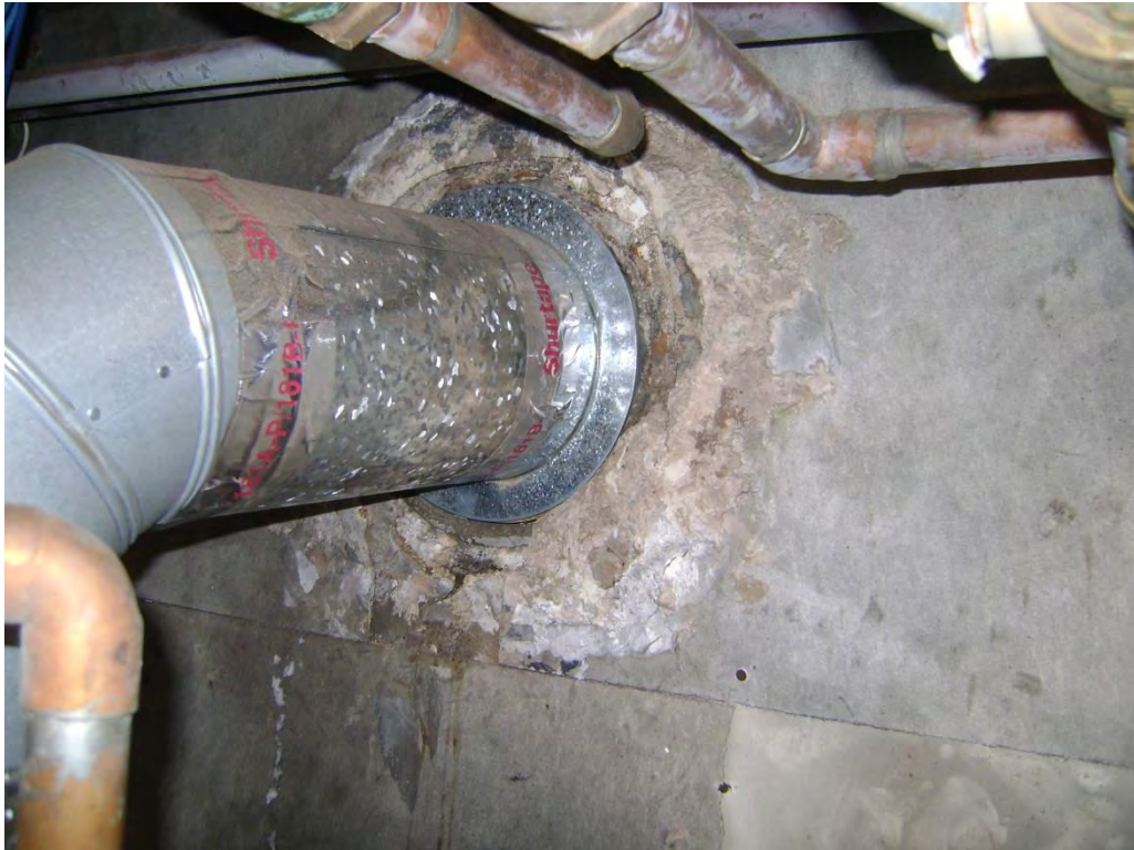
Sample #228 - Flue Sealant - 1.75% Chrysotile
