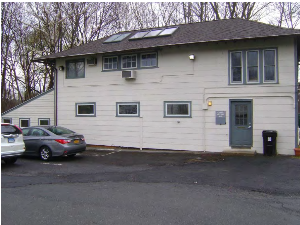
Sample #246 - Cementitious Siding - 33.30% Chrysotile
