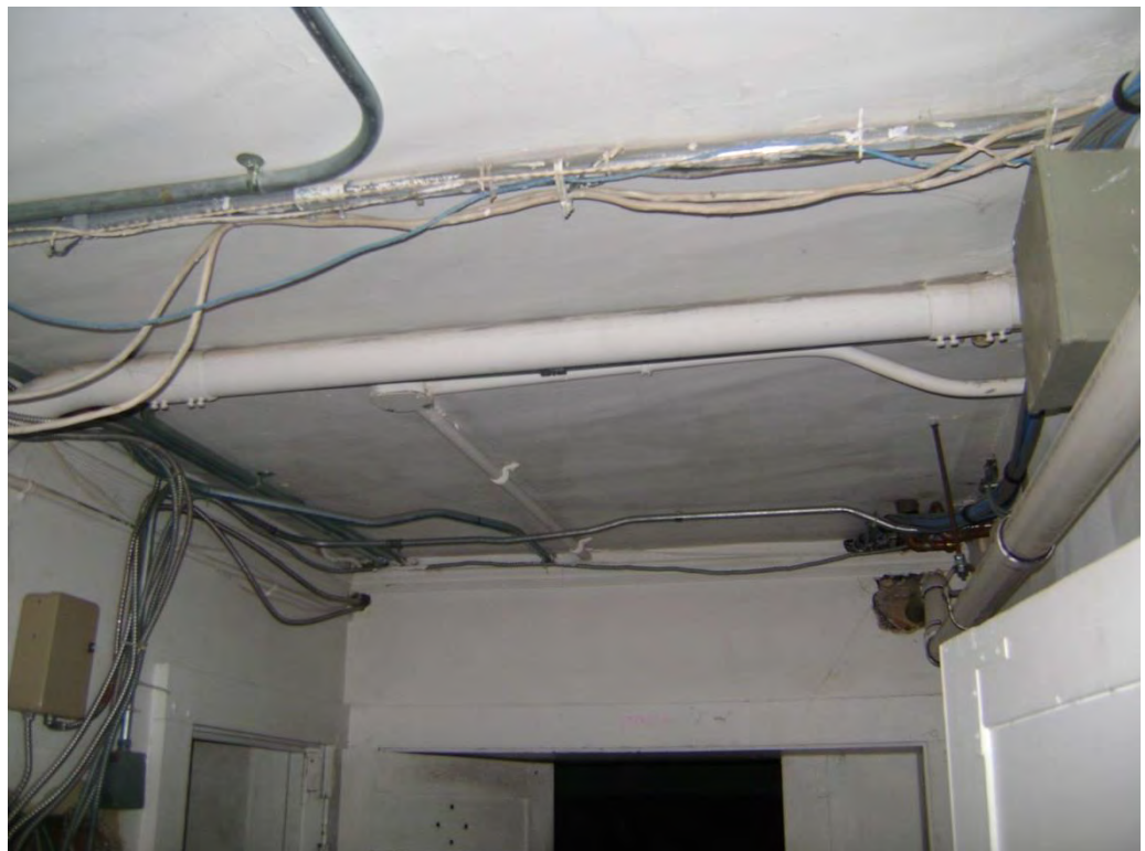
Sample #24 – Plaster Ceiling Base Coat – 1.54% Chrysotile
