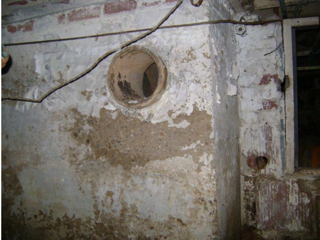
Sample #211 – Flue Sealant – 1.4% Chrysotile
