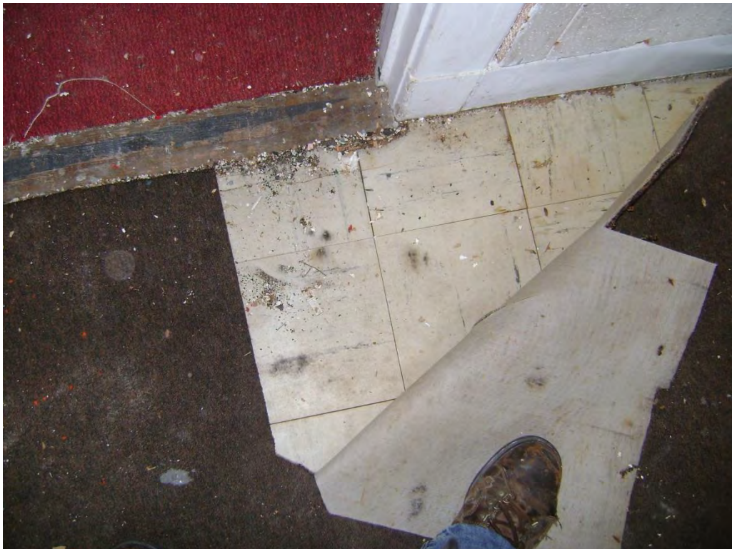
Sample #212 – 9x9 Floor Tile and Mastic – 1.2% Chrysotile
