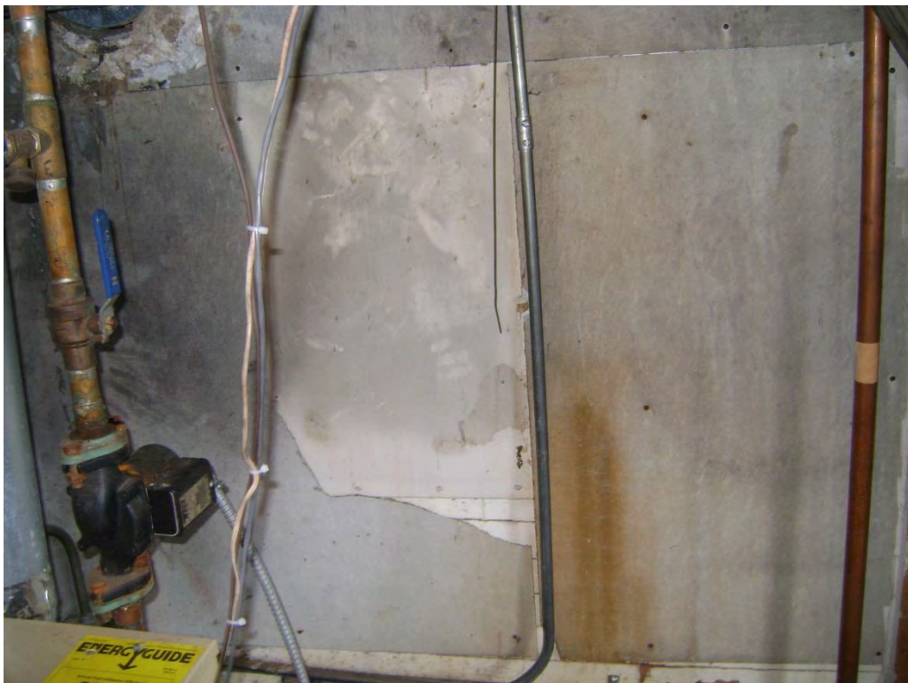
Sample #226 – Cement Board – 36.40% Chrysotile
