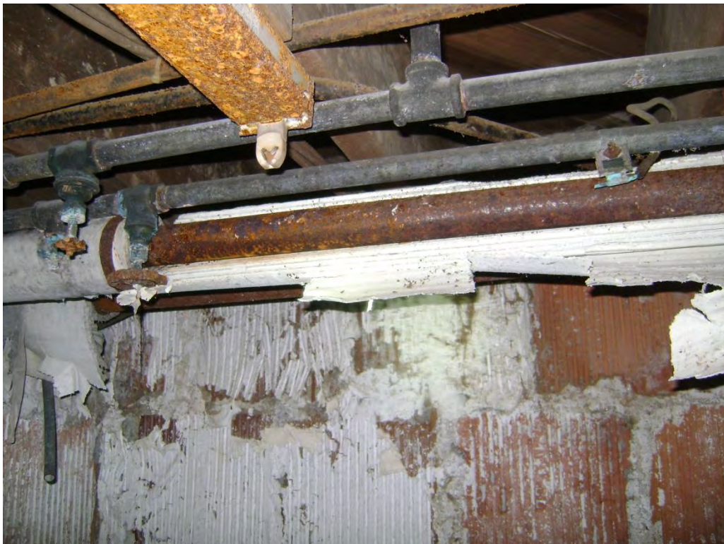
Sample #202 and 205 – Pipe Insulation and Mudded Fitting – 80.00% and 40.00% Chrysotile
