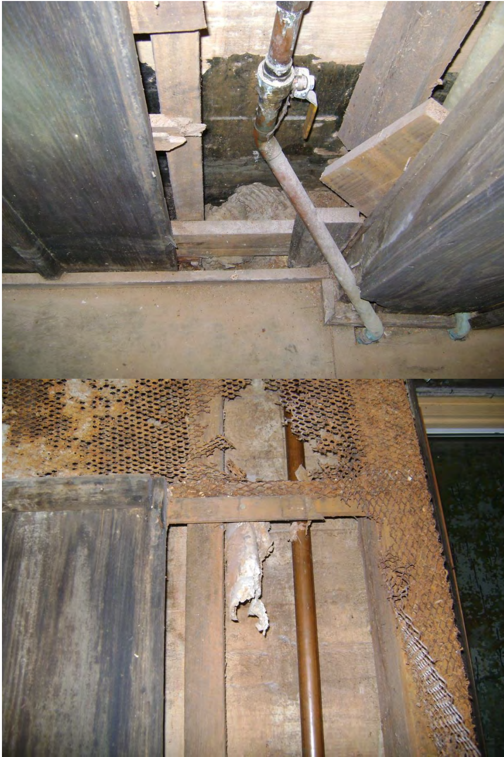
Sample #52 - Pipe Insulation Debris - 19.10% Chrysotile
