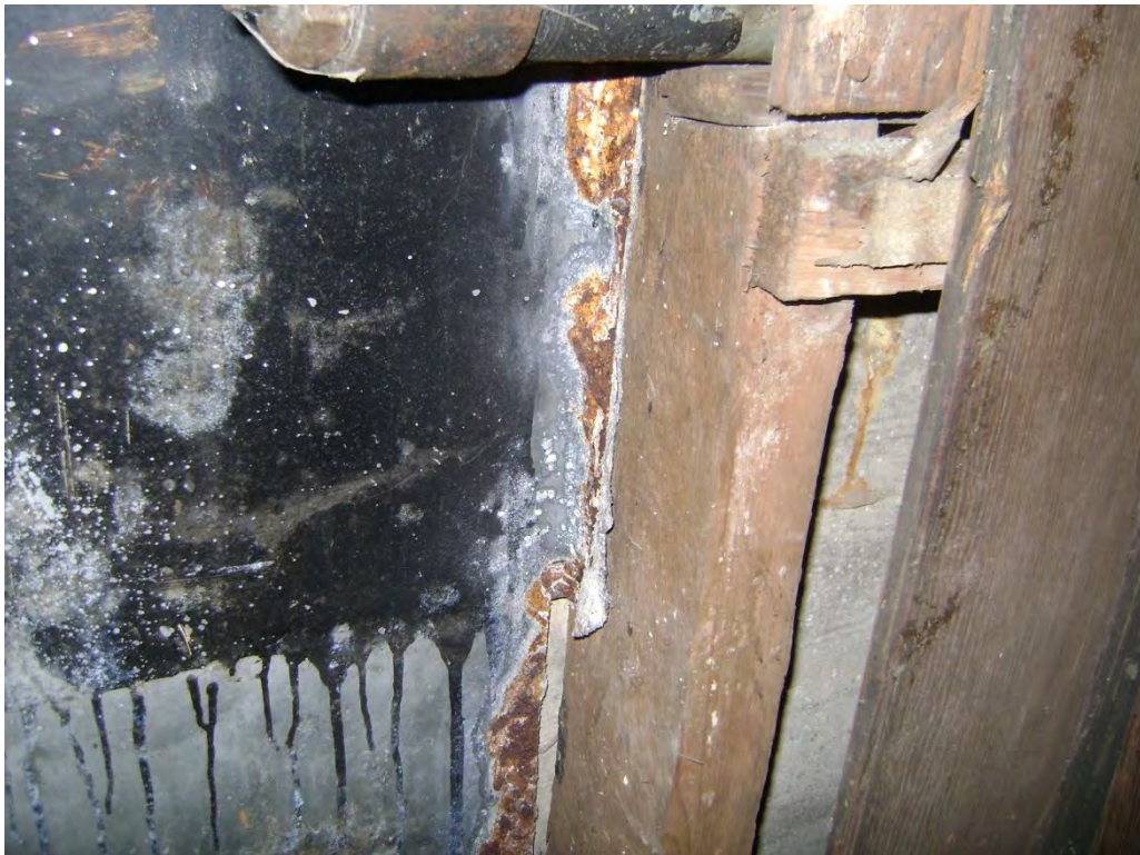
Sample #49 – Material Behind Heat Shield – 50% Chrysotile
